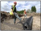
**BasaMesh<sup>™</sup> for Paving:** Used for reinforcing road and highway asphalt overlays to prolong the pavement's lifespan by reducing the effects of reflective cracking caused by traffic loading, age hardening, rutting, shoving and temperature cycling. Pavement life between maintenance intervals is also significantly extended. Basalt reinforcing mesh makes it possible to reduce the thickness of asphalt pavement up to 20% when combined with BasaMix<sup>™</sup>.
